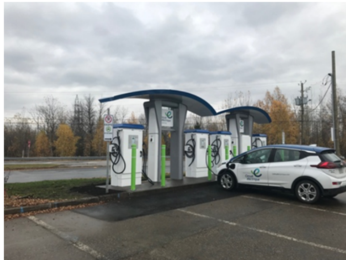
Figure 1. The superstation (source HQ web site)
